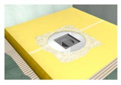
It is prepared by cutting butyl tape in appropriate sizes around the shower channel, strainer or drain unit.
