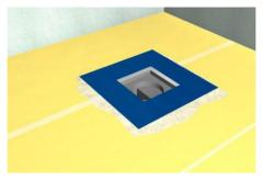
Step 3 After the surface preparation is completed, the shower channel, strainer is placed on the floor and the butyl tape is adhered to the floor and it is ensured that it is well adhered to the floor on which it is applied with a pressure roller.
